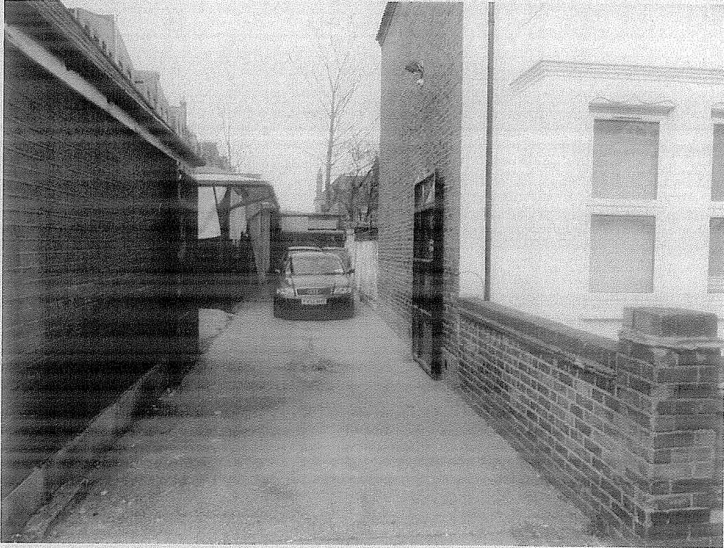
Below: the gates of the alleyway. On the right 1 Stanhope Gardens.
